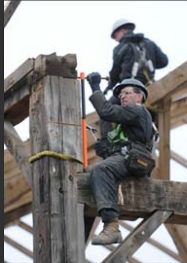
Deconstruction of Harts Lane barn
